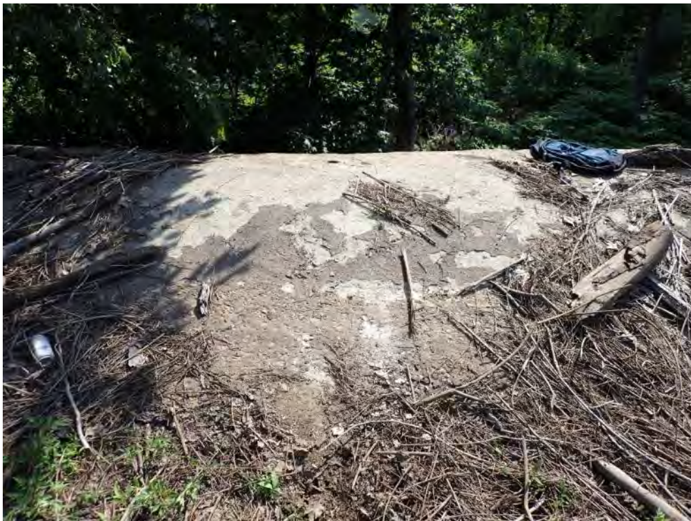
Photo 16 – View of spillway crest (7/10/2019)
