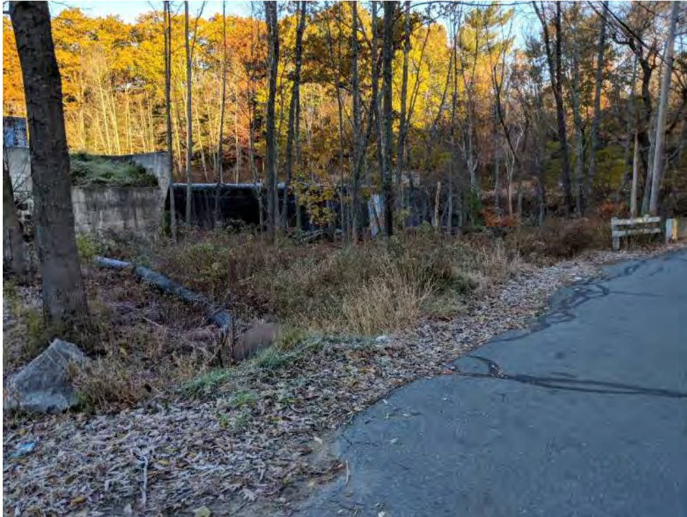
Photo 3 – Overview of spillway from downstream (11/08/2018)
