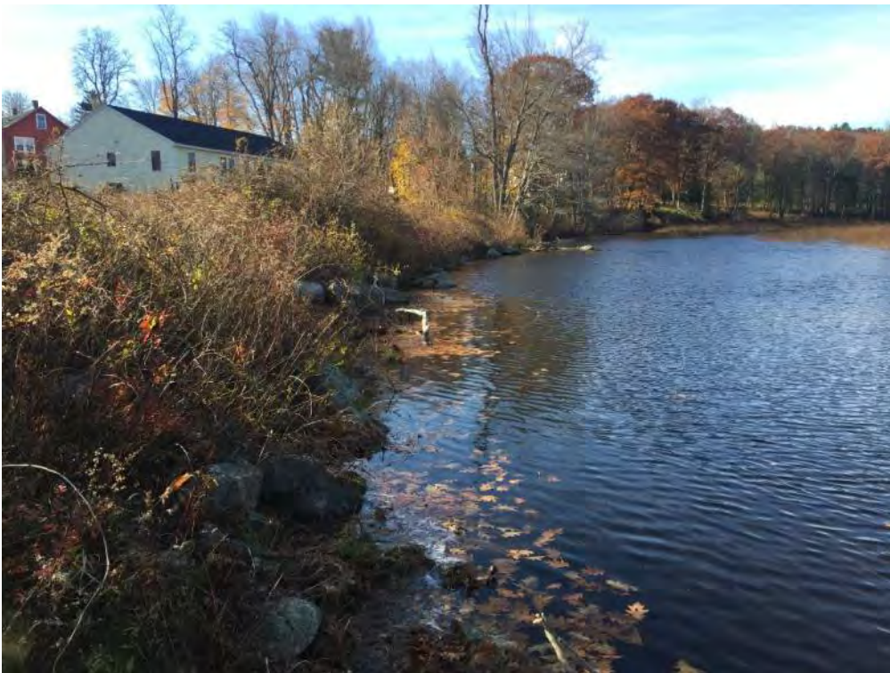
Photo 35 – Upstream slope of embankment looking right (11/8/2018)
