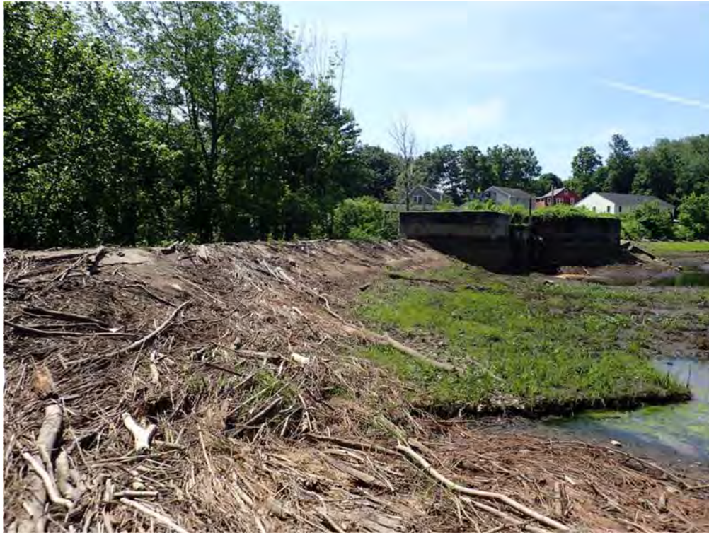
Photo 15 – Overview of spillway from left side (7/10/2019)
