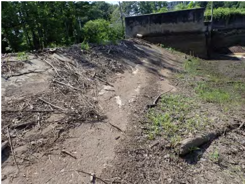
Photo 18 – View of spillway crest looking right (7/10/2019)
