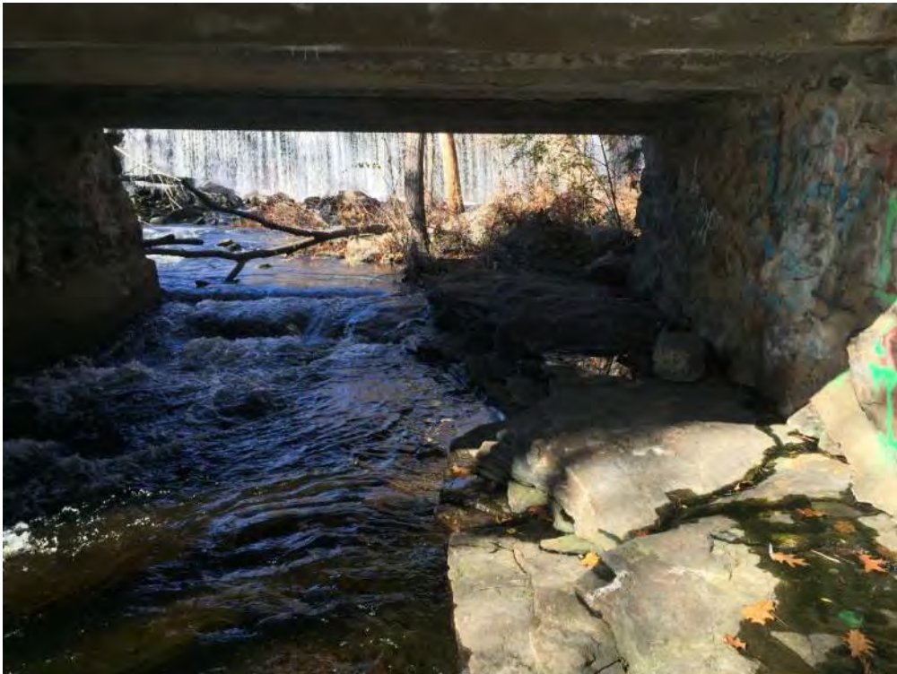
Photo 42 – View through north bay of Sanborn Street bridge; note weir at inlet (11/8/2018)
