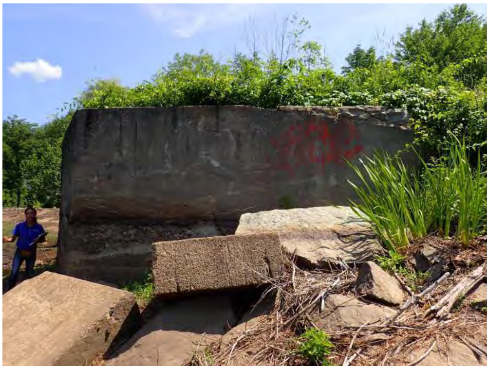
Photo 25 – Right section of right upstream wall (7/10/2019)
