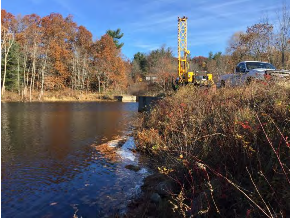
Photo 36 – Upstream slope of embankment looking left (11/8/2018)
