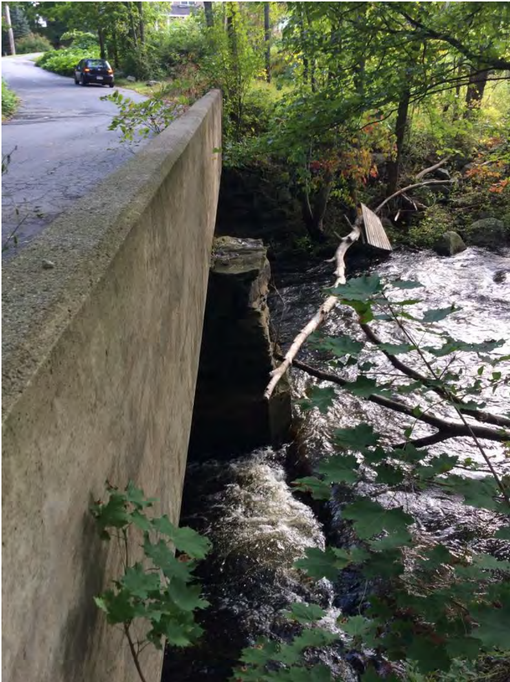
Photo 40 – Weir at inlet of Sanborn Street Bridge (11/8/2018)
