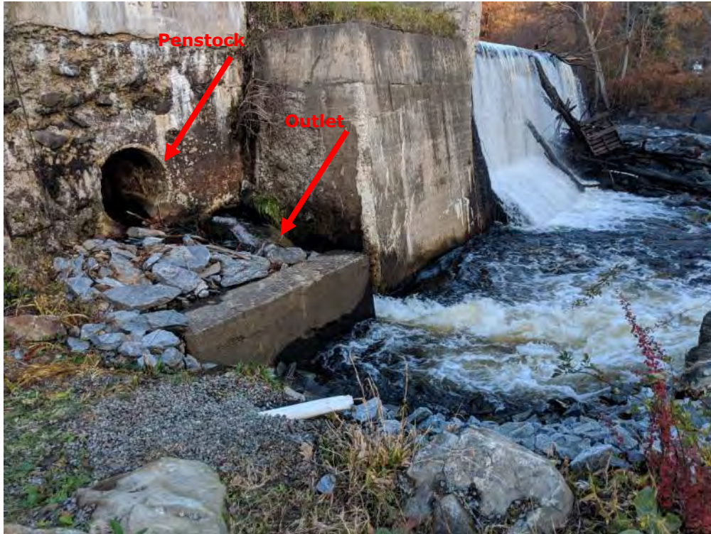
Photo 5 – Former penstock outlet and low-level outlet (11/08/2018)
