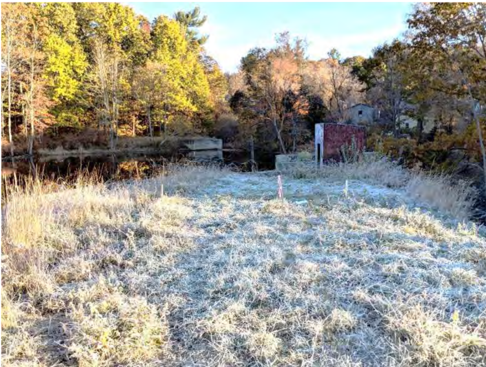
Photo 10 – Embankment crest from right abutment (11/8/2018)
