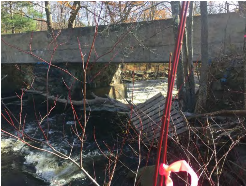
Photo 39 – Inlet of Sanborn Street Bridge (11/8/2018)
