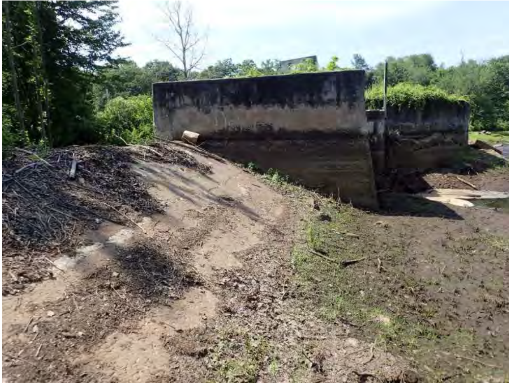
Photo 19 – Overview of right training wall (7/10/2019)
