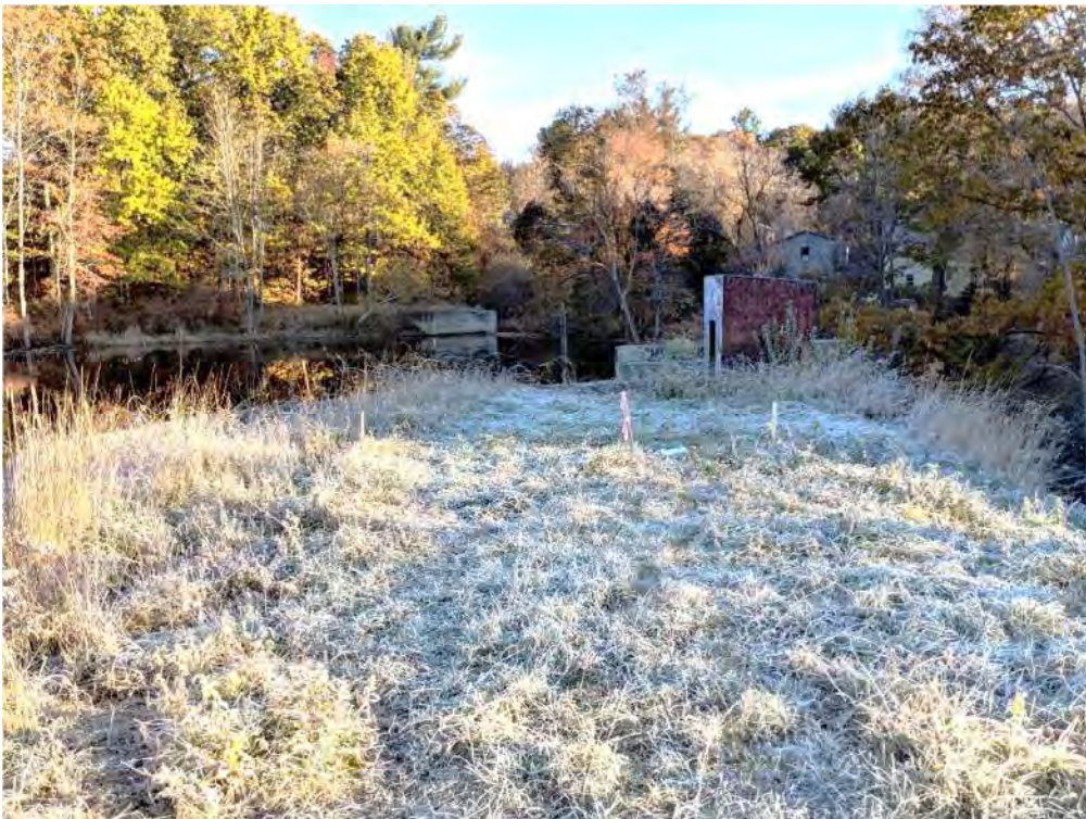
Photo 10 – Embankment crest from right abutment (11/8/2018)
