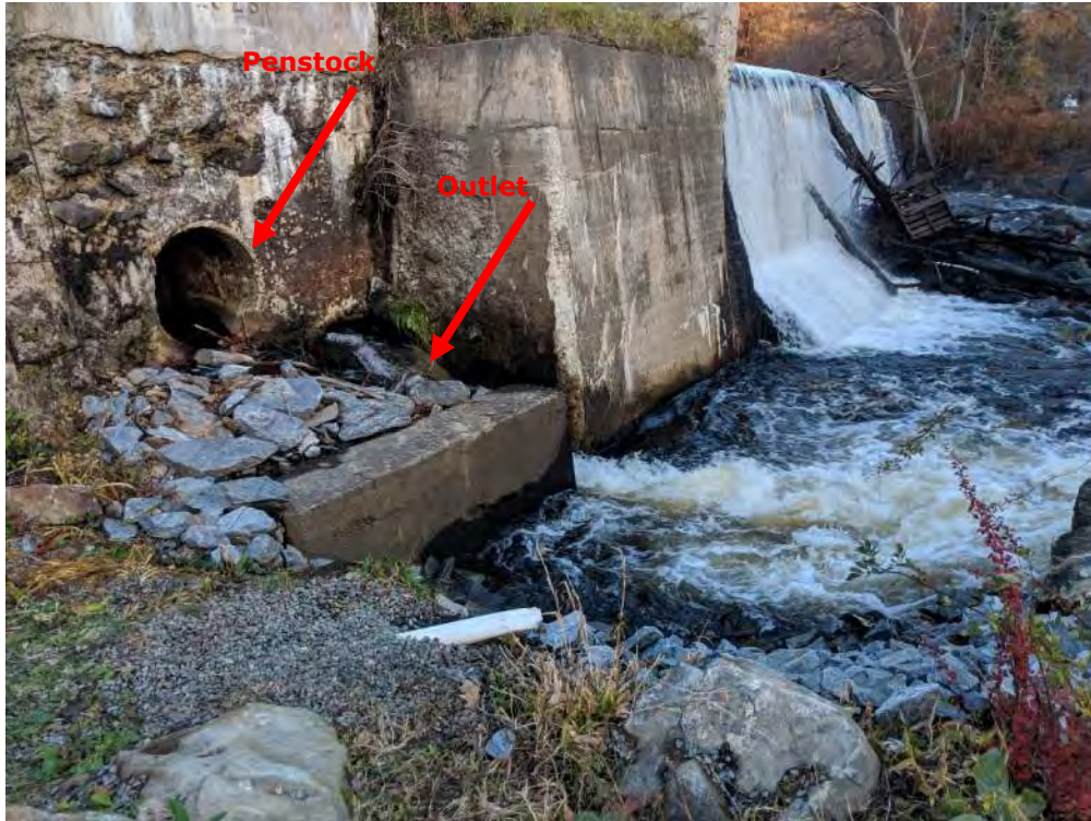
Photo 5 – Former penstock outlet and low-level outlet (11/08/2018)
