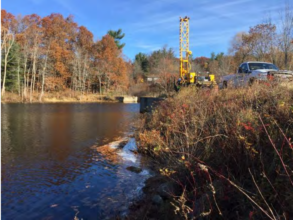
Photo 36 – Upstream slope of embankment looking left (11/8/2018)
