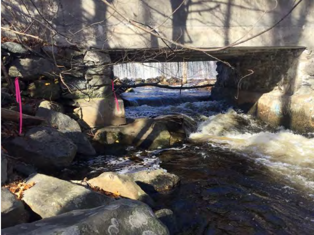
Photo 41 – View through south bay of Sanborn Street bridge; note weir at inlet (11/8/2018)
