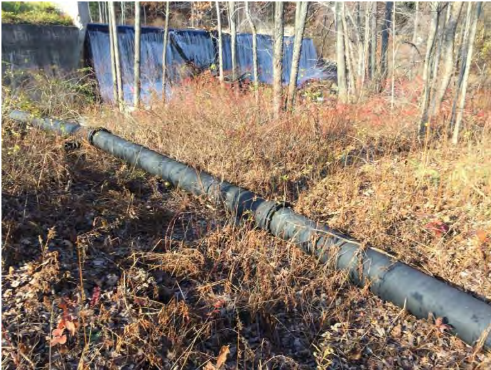
Photo 38 – Former penstock pipeline, surrounded by wetland flag series 1D (11/8/2018)
