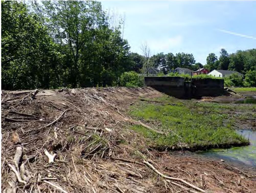
Photo 15 – Overview of spillway from left side (7/10/2019)
