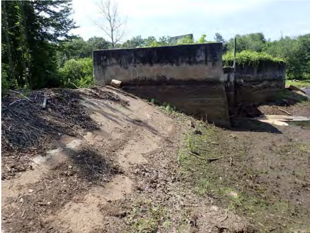
Photo 19 – Overview of right training wall (7/10/2019)
