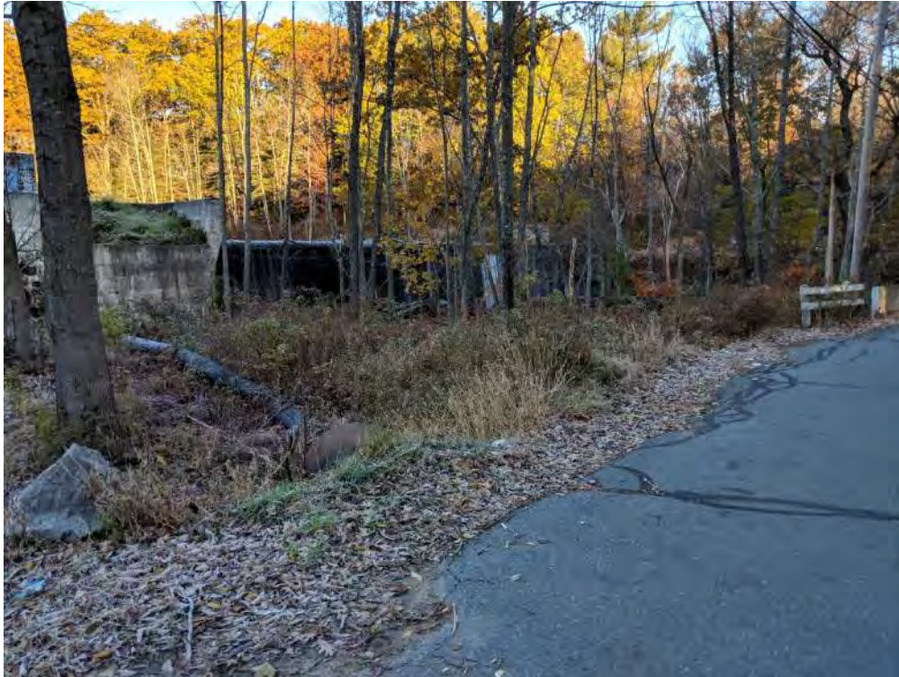
Photo 3 – Overview of spillway from downstream (11/08/2018)
