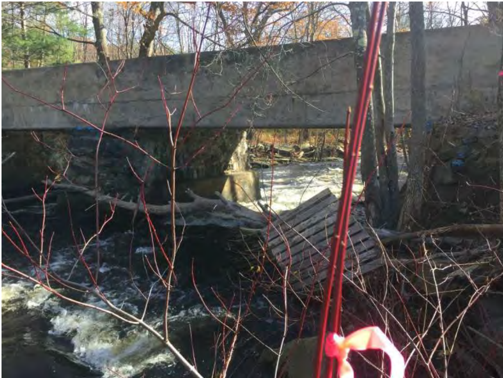
Photo 39 – Inlet of Sanborn Street Bridge (11/8/2018)
