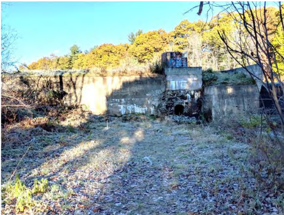
Photo 4 – Overview of outlet structure and right downstream wall from downstream (11/8/2018)
