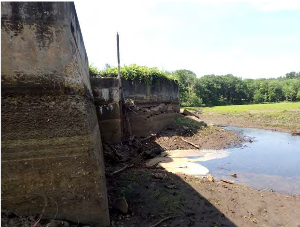
Photo 22 – Overview of upstream side of right embankment showing stream entering outlet (7/10/2019)
