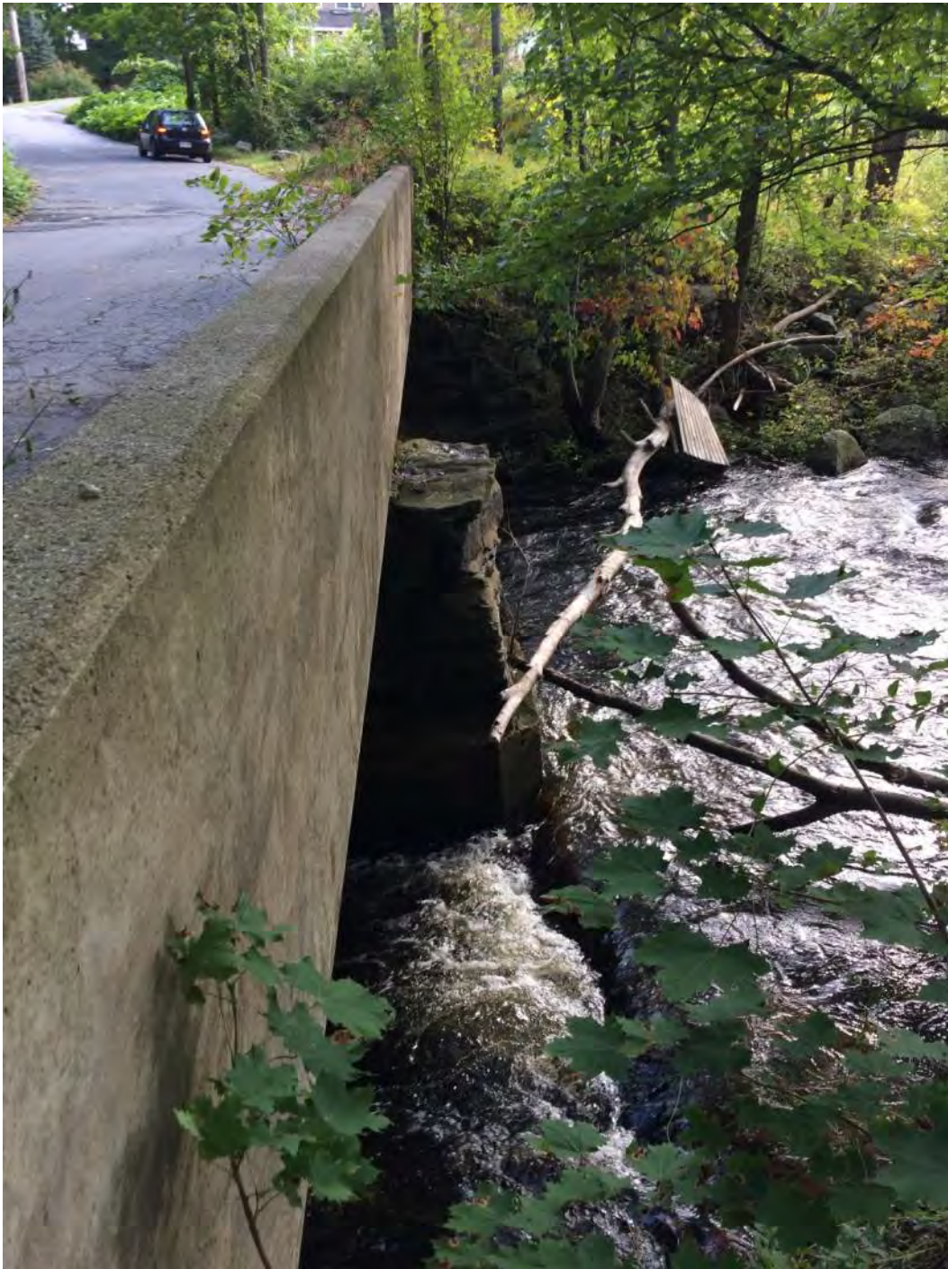
Photo 40 – Weir at inlet of Sanborn Street Bridge (11/8/2018)
