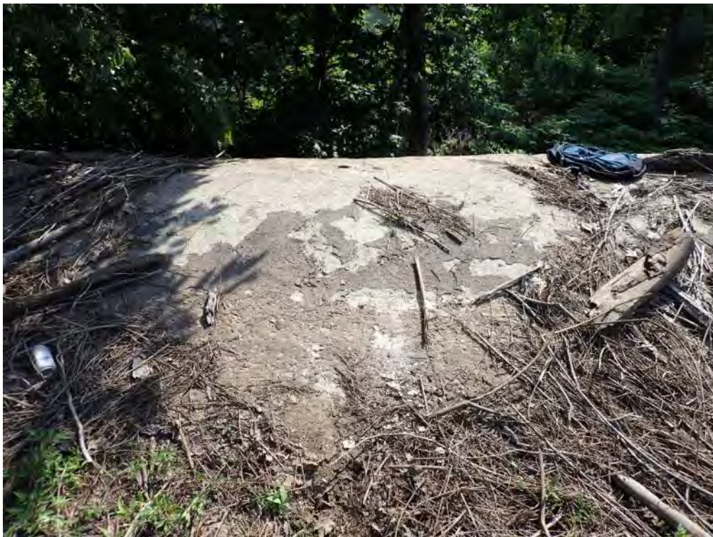
Photo 16 – View of spillway crest (7/10/2019)
