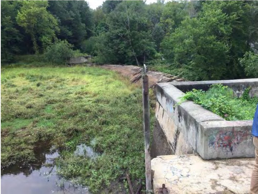
Photo 7 – Overview of spillway from upstream (9/13/2018)
