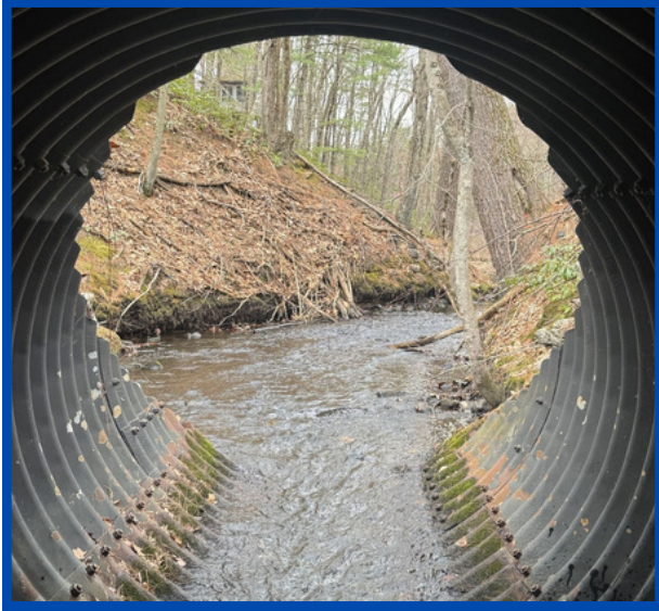
Figure 6: 7 foot round metal culvert. Stream Crossing group 2026.
