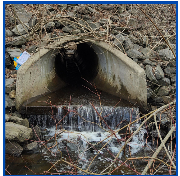
Figure 15: A round culvert that free falls into cascade. Stream Crossing group 2026.
