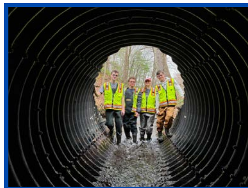
Figure 1: Stream crossings team inside of 7 foot round metal culvert
