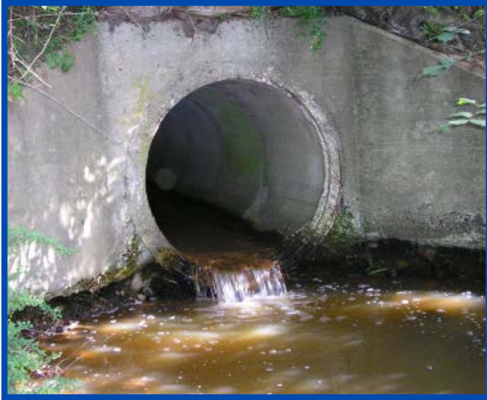
Figure 8: Round concrete culvert outlet with headwall, wingwalls, free fall, and scour pool (NAACC, 2019)
