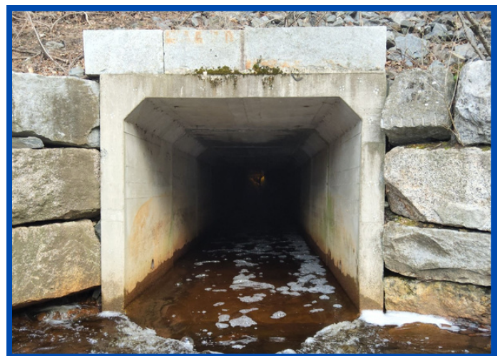
Figure 2: 7 foot concrete box culvert in Pepperell MA
