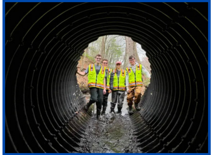
Figure 16: Our group investigating a culvert during assessments. Stream Crossing group 2026.
